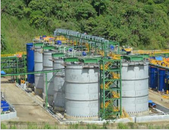
FIGURE 3 - AGITATED CYANIDE PLANT
